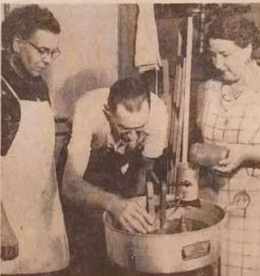
HOW TO CUT A GEM—With Mrs. Maurice Tracy (left) and Mrs. K. F. Dodge (right) as onlookers, Lincoln Mineral and Gem Society President Maurice Tracy cuts a piece of yellow jasper picked up in a limestone quarry near Garland. Mrs. Dodge is pouring oil on the diamond edged cutting wheel.
